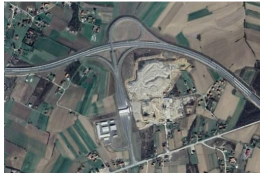
Figure 11b. Highway build up (2018)
